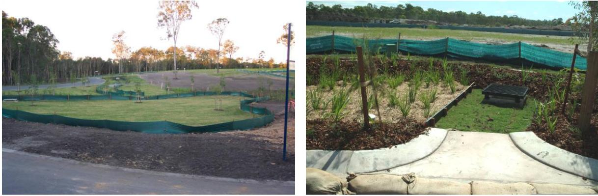
Figure 2. Protection of filter media with a geofabric and turf cover (left) and use of a sacrificial sediment forebay during construction and plant establishment (right).
